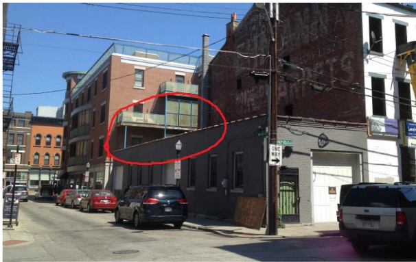
EXISTING FROM NORTHWEST CORNER AT 14TH AND REPUBLIC
